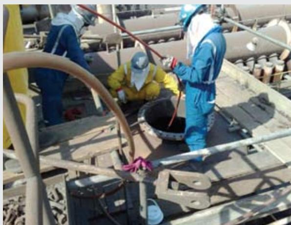
Preheater tube bundle cleaning by hydro-jetting in progress
